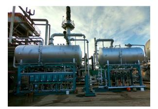
SKID-MOUNTED UNITS Figure 3. Installing these two high-pressure, skid-mounted deaerators rental units required cranes for offloading and placing at the jobsite.
