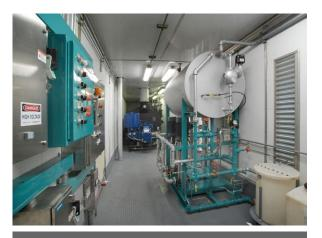
INTERNAL VIEW OF MOBILE BOILER ROOM Figure 1. This trailer-enclosed mobile boiler room contains a fire tube boiler and all necessary auxiliary equipment.
