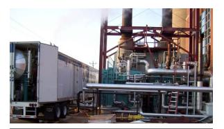
FEEDWATER TRAILER Figure 6. This application required temporary installation of two 82,500-lb/hr boilers and a mobile feedwater trailer.
