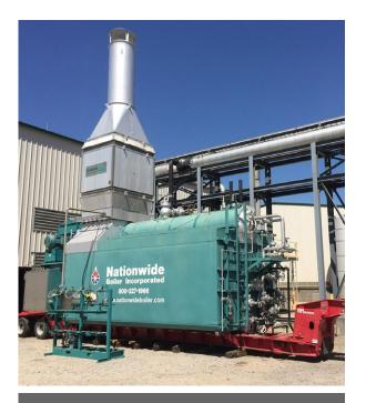
NOX COMPLIANCE Figure 8. This application required temporary installation of one trailer-mounted package water tube boiler and CataStak SCR system for sub 5ppm NOx compliance.
