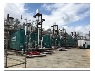
MULTIPLE BOILERS INSTALLED IN PARALLEL Figure 5. Five 75,000 lb/hr trailer-mounted superheated steam boilers with Urea-based CataStak selective catalytic reduction systems are installed in parallel.
