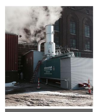
WEATHERPROOF ENCLOSURE Figure 7. This package water tube rental boiler includes a temporary enclosure for temperature conditions at or below freezing.
