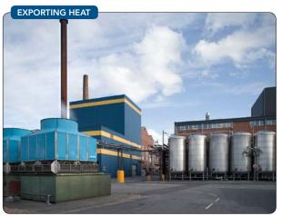
Figure 2. Grinsted plant in Denmark no longer rejects surplus heat but instead sends it to a district heating company. Source: DuPont.
